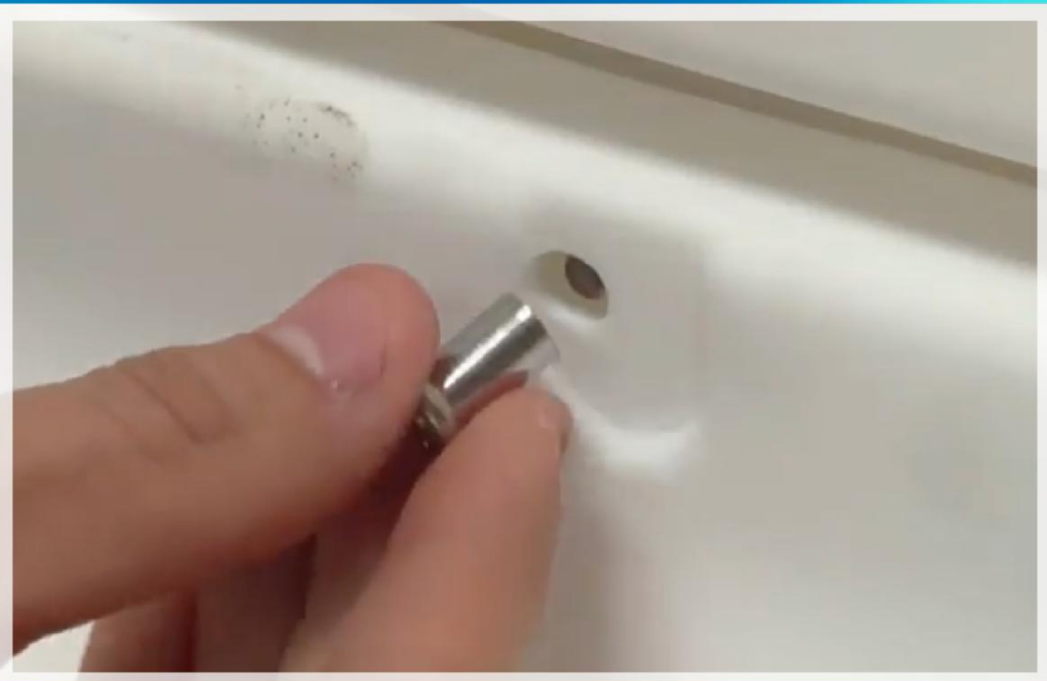
Secure it on the opposite end with the barrel nut.
