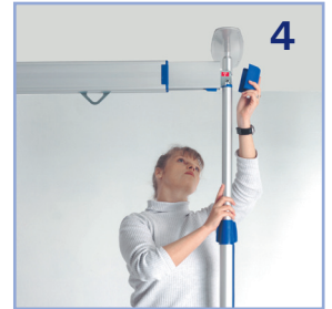
Fix the end cap to lock the rail in place.
