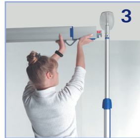
Extend the rail to required length and fix the rail onto the second post.
