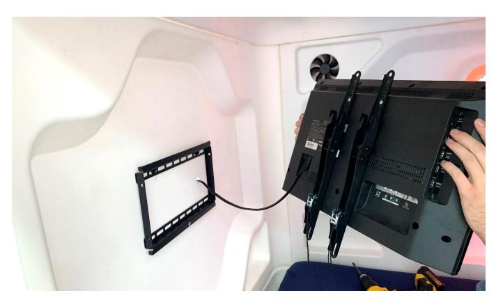
Step 15. Use the hooks on the braces to mount the TV on the bracket. Adjust as needed and your TV is now installed!
