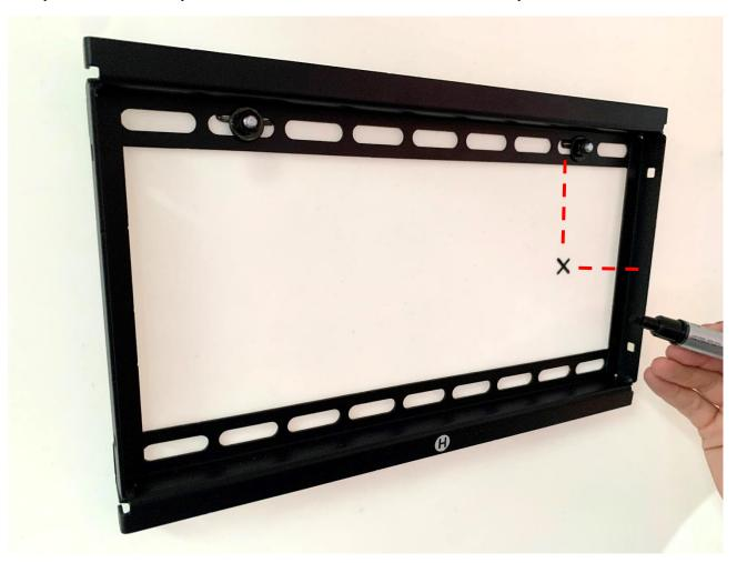
Step 13. Drill a hole COMPLETELY through the mark you just made. Use the drill bit to widen the hole enough for the smaller end of the TV power cable to fit through.
