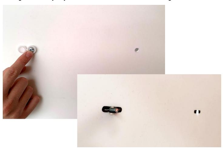
Step 6. Place a washer and a nut over the bolt.
