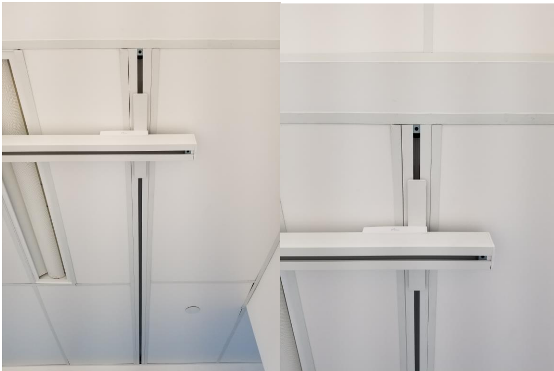
Figure 4: Physical example of the final look of an installed recessed track
