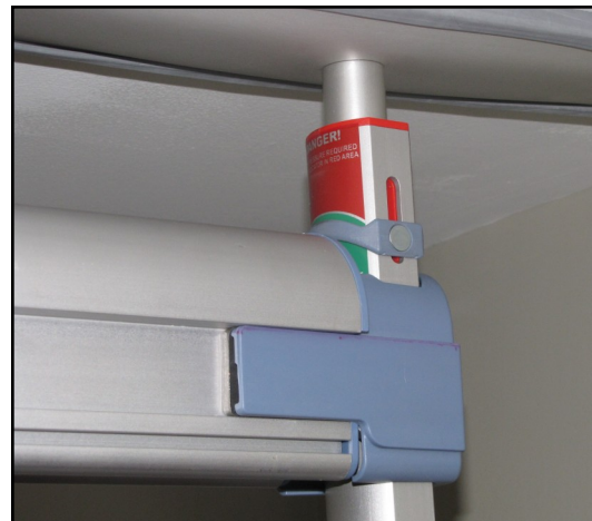
Step 14b: Install the other end cap.
