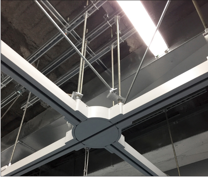
Typical turntable installation with Unistrut hardware and ½" (12.7 mm) threaded rods.
