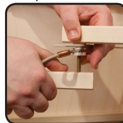
Remove wood brace
