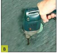
Drill a 7/16" hole completely through the floor board as shown in Figures B and C.
