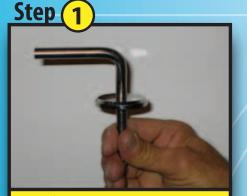
Screw flanges all the way up so that there are no threads showing
