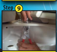
Secure the seat using pliers... DO NOT OVER TIGHTEN.
