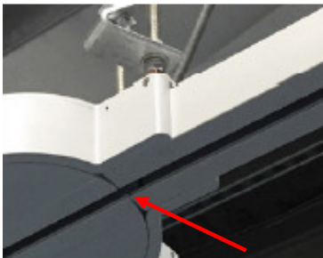
Figure 16 – File the edges of the track
