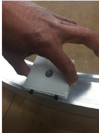
Figure 12 – Note orientation of ceiling brackets
