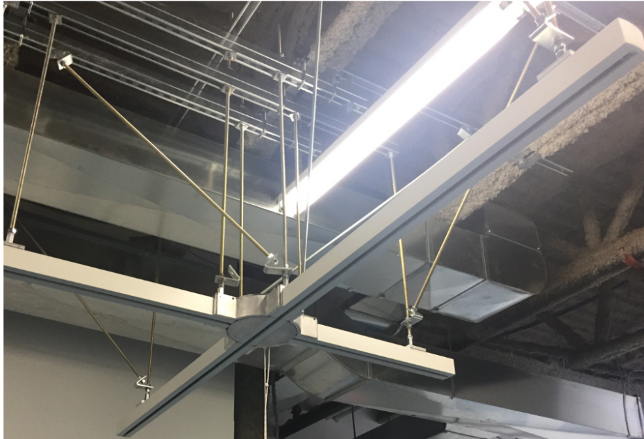
Typical turntable installation with Unistrut hardware and 1/2" threaded rods.
