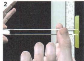
Hold ends of straps between thumb and forefinger and pull toward you until channel rests flush behind wall. Slide plastic cap along straps with other hand until flange of cap is flush with wall.
