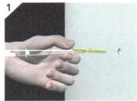
Drill a 1/2" ( $\varnothing$ 13mm) hole. Hold metal channel flange alongside plastic straps and slide channel through hole. Minimum clearance behind wall: 1-7/8" (48mm).
