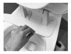
Holding the bidet attachment in place, tighten the Stay•Tite nuts until the installation head snaps off.
