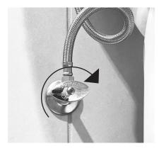
Close the water supply valve to the toilet. Flush the toilet to minimize the water in the tank. Place a towel on the floor to absorb any water.
