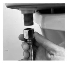
2. Disconnect the water hose from the fill valve connection under the tank of the toilet.
