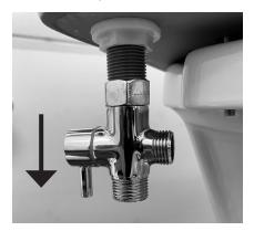
Confirm that the rubber washer is in the t-valve. Connect the adjustable t-valve to the underside of the toilet tank. Turn the water control handle downwards. This shuts off the water to the bidet attachment.
